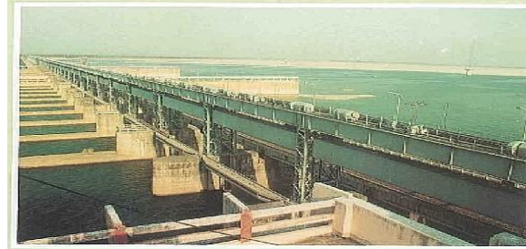
A project of national-level importance, being the terminal barrage on the river Ganges, located in the state of West Bengal, completed in 1974, serves the purpose of flushing the channels of Calcutta Port, as well as to augment water supply to Calcutta city.
